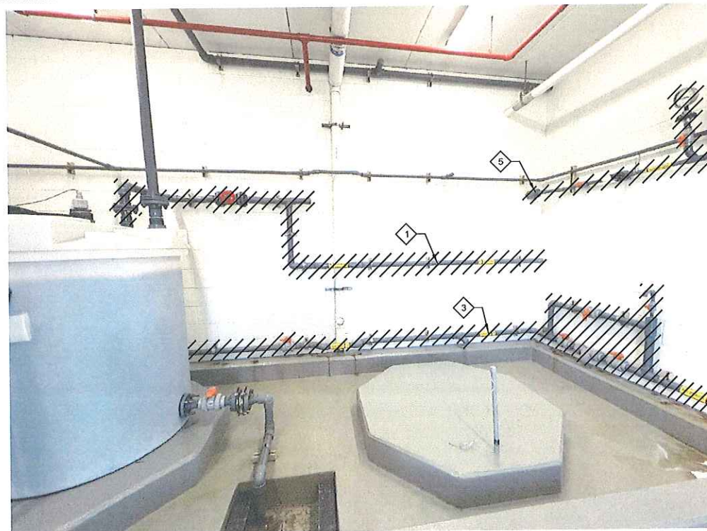
SULFURIC ACID BULK STORAGE TRANSFER
